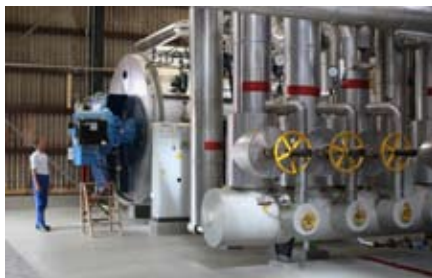
Hydrogen boiler, Cheminova DK.
